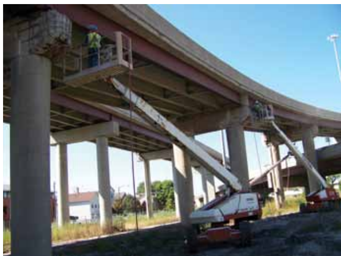
This elevated structure runs through the heart of the city of Chicago
