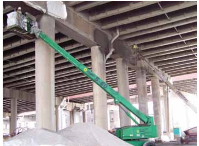
Use of shotcrete over form and pour was chosen for its advantages in "green building"
