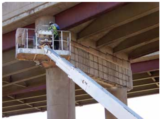
120 piers approximately 60 ft (18.28 m) high above local roads, businesses, and railways
